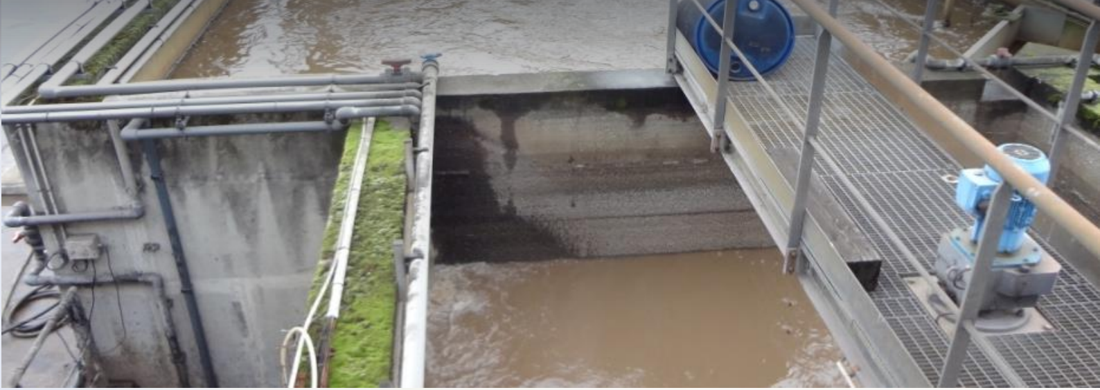
Settling ponds of Tank service Saint Pol sur mer (France, 59) facility.
